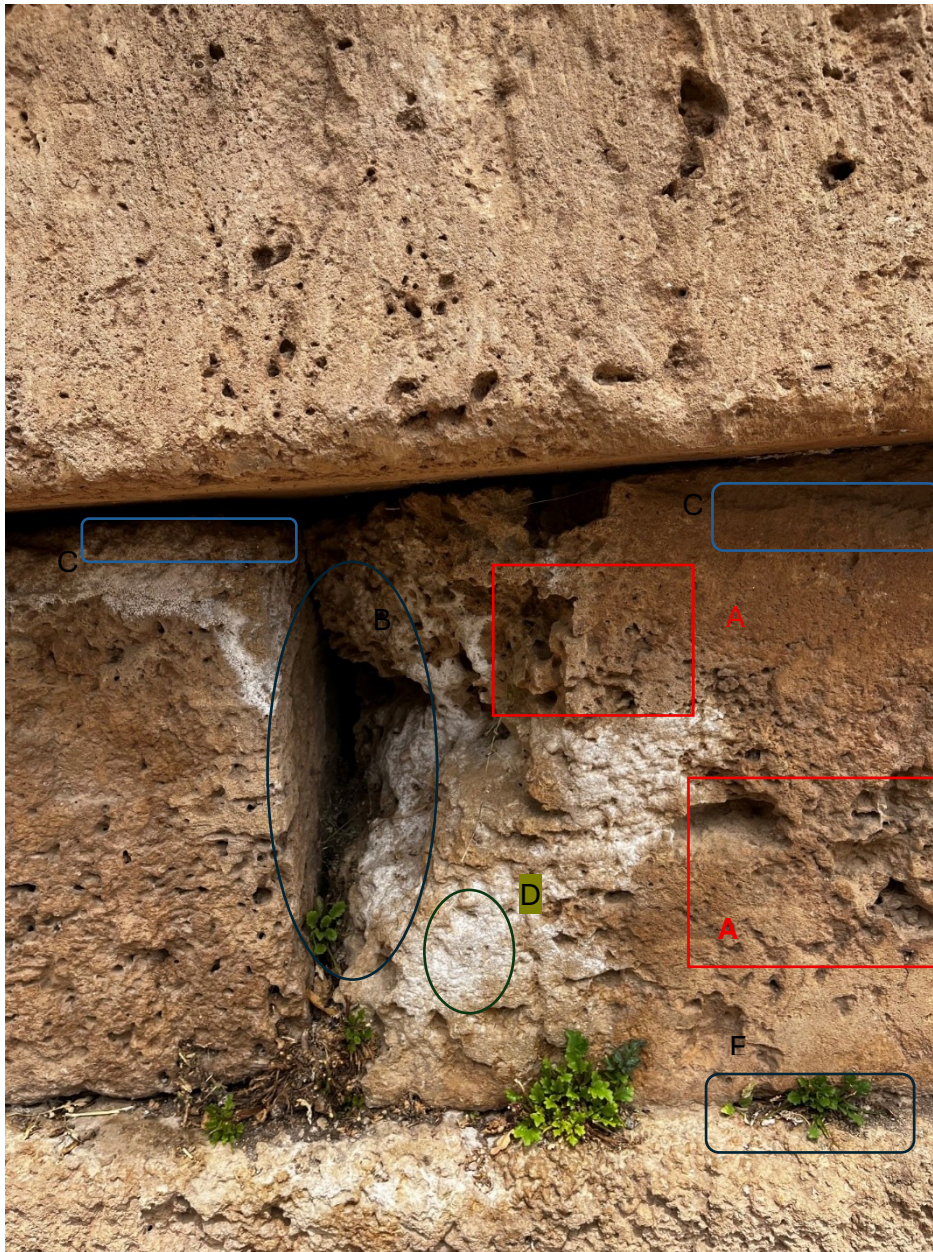
Figure 8. Deterioration patterns observed on a stone element of the Temple of Apollo: (A) alveolar weathering, (B) material loss and surface recession, (C) differential erosion and rounding, (D) white surface deposits possibly associated with salts, and (E) higher plant growth, identified macroscopically according to the ICOMOS–ISCS (2008) terminology (author’s photograph, 2026).
