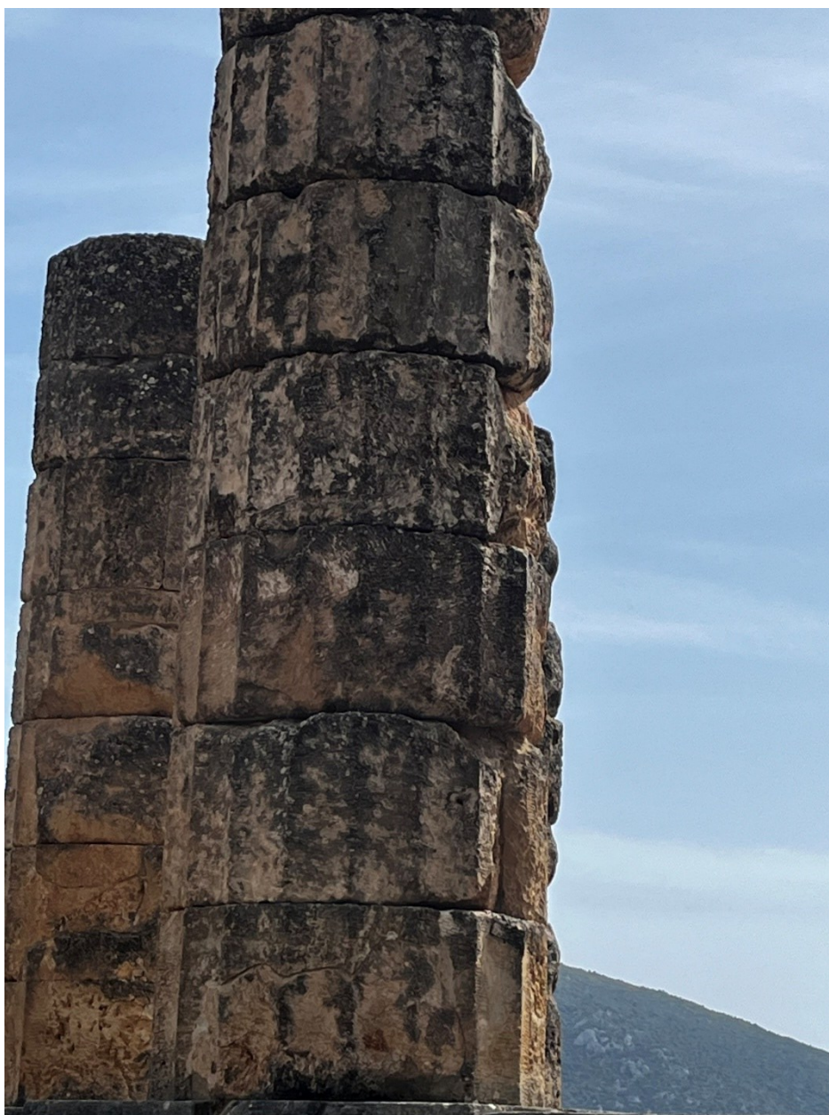
Figure 13. General view of discoloration and surface deposits on stone elements of the Temple of Apollo, with visible cracks, discontinuities and rounding of stone edges (author's photograph, 2026).
