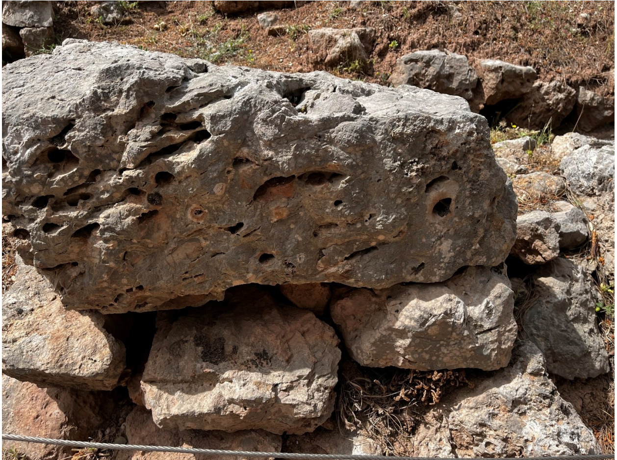
Figure 19. Pronounced alveolization in a stone element in the area of the Ancient Stadium of Delphi, characterized by the development of multiple cavities and localised material loss on the stone surface. The deterioration pattern was identified macroscopically according to the ICOMOS–ISCS (2008) terminology, (author’s photograph, 2026).
