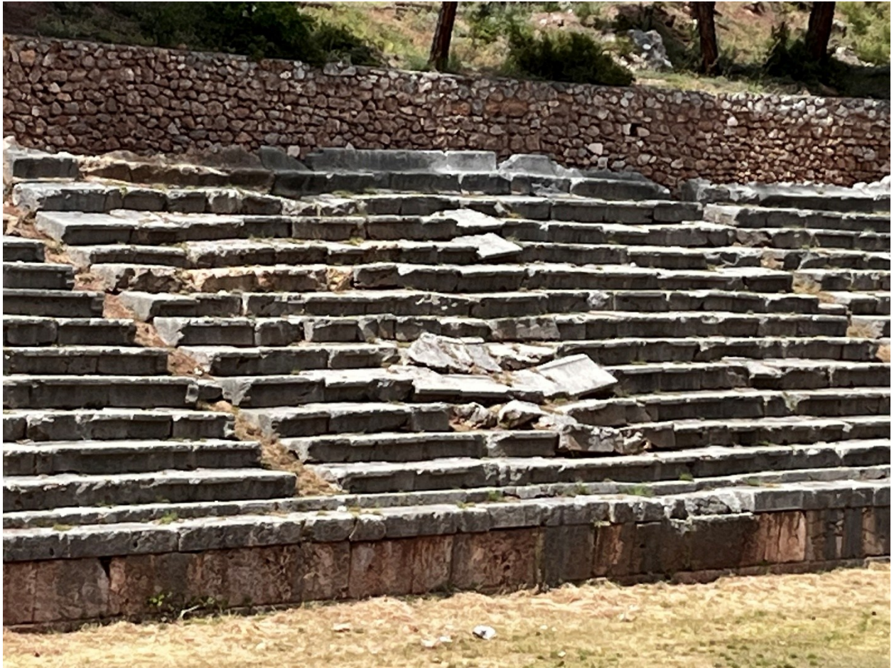
Figure 16. Extensive disorganisation and localised displacement of stone elements in the seating tiers of the Ancient Stadium of Delphi, with detached stone fragments present in the central area. These observations document the macroscopic condition of the seating tiers, while visual examination alone does not allow the mechanisms or factors that led to the observed condition to be determined (author's photograph, 2026).
