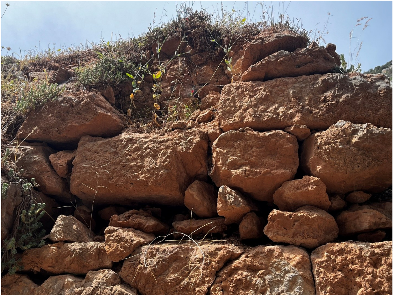
Figure 17. Stone elements and vegetation on the slope in the area of the Ancient Stadium of Delphi. The localised removal of loose soil material may be associated with surface runoff and washing by water, although this mechanism cannot be confirmed through visual observation alone. The presence of plants is recorded as biological colonisation (plant), according to the ICOMOS–ISCS (2008) terminology (author’s photograph, 2026).
