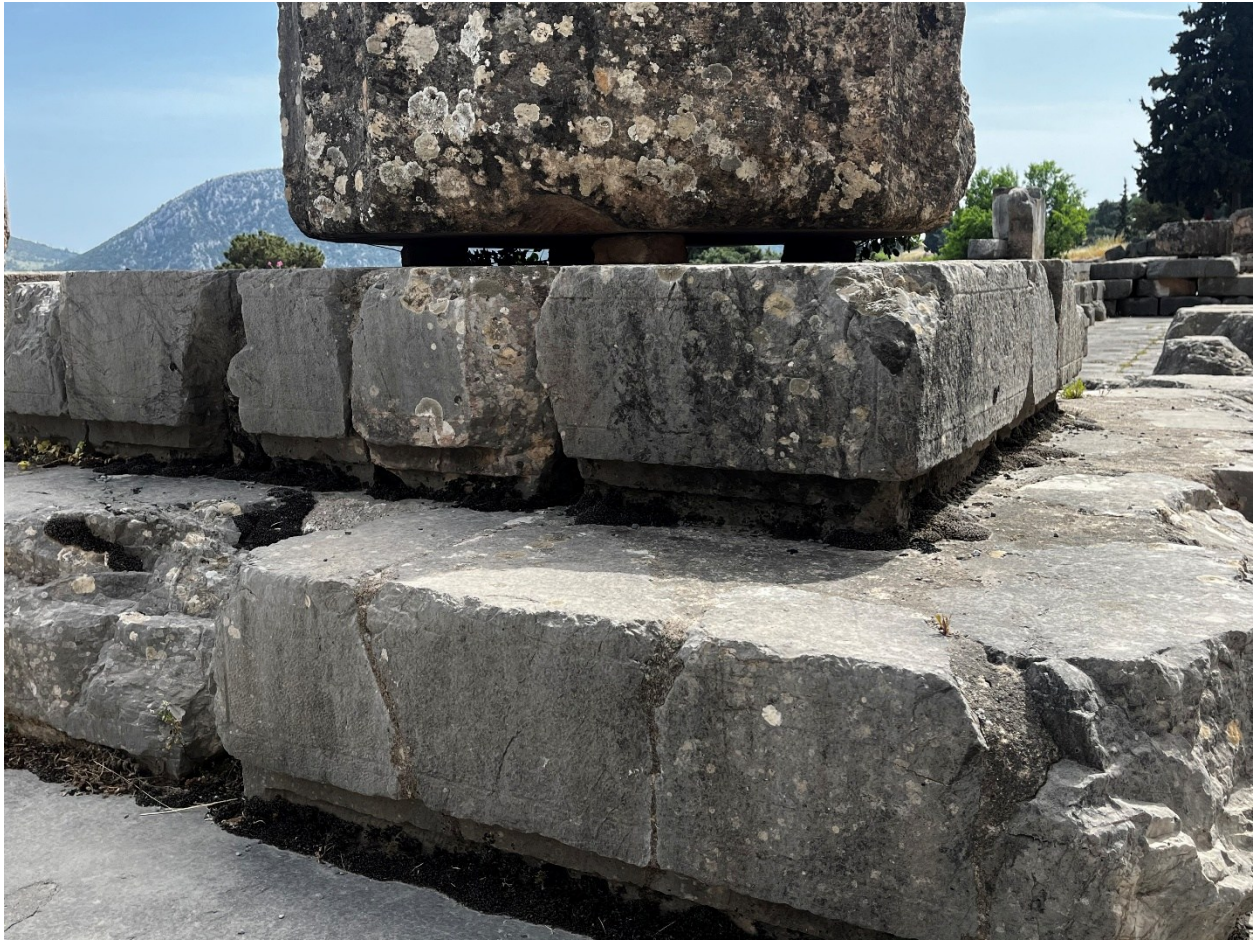
Figure 12. Lichen colonisation and biological surface deposits observed on an architectural element of the Temple of Apollo.
