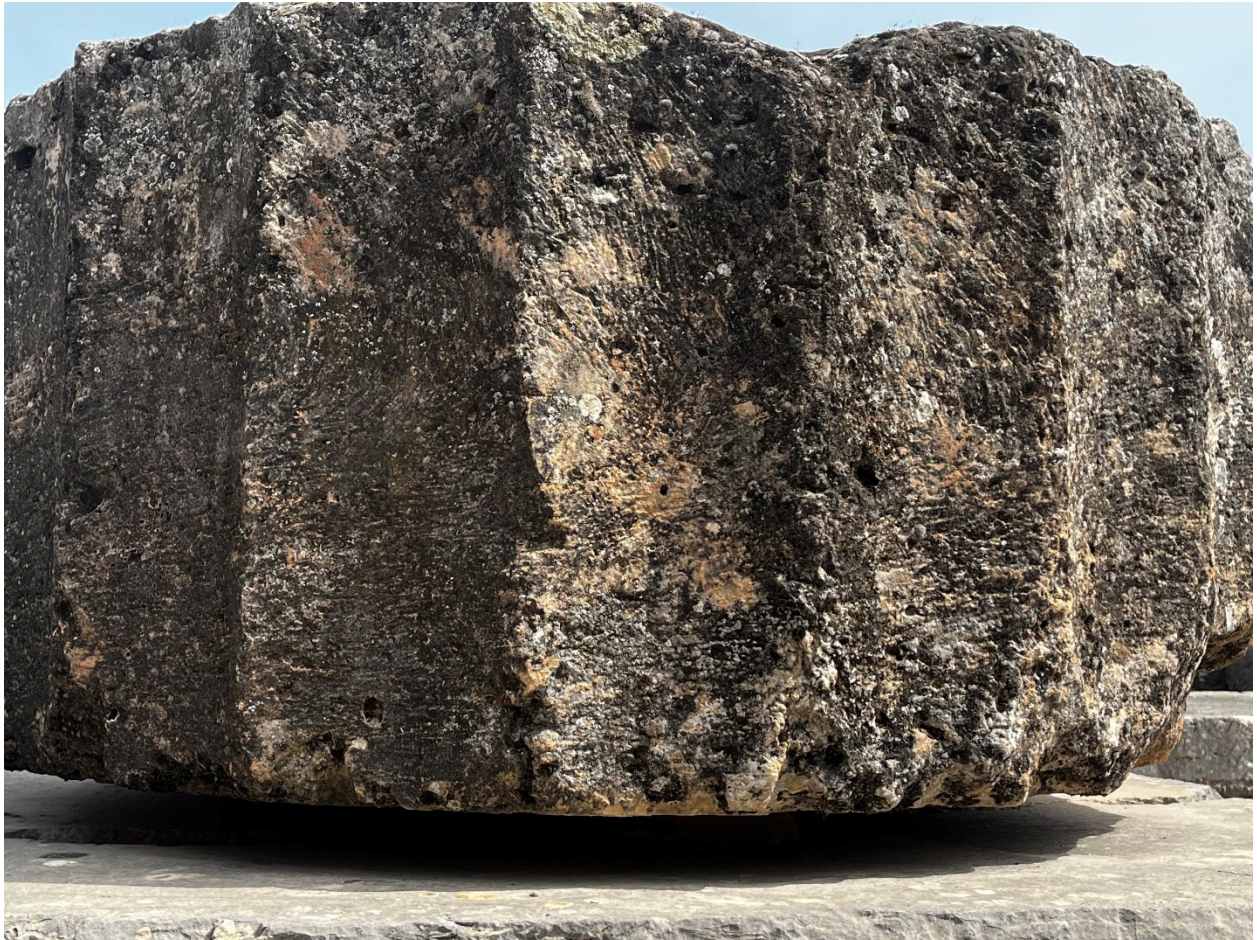
Figure 7. Deterioration patterns observed on a column drum of the Temple of Apollo, including alveolarization, rounding of the stone edges, and biological colonization, identified macroscopically according to the ICOMOS-ISCS (2008) terminology (author's photograph, 2026).
