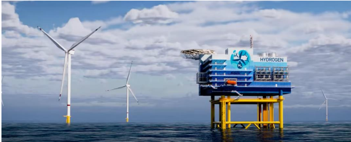
Figure 42: AquaVentus project (3D presentation) coupling offshore wind with hydrogen production
