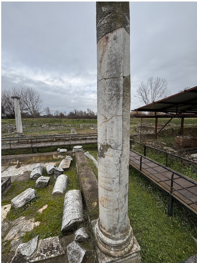
Figure 4.41: Penetration of vegetation into masonry (personal archive).
