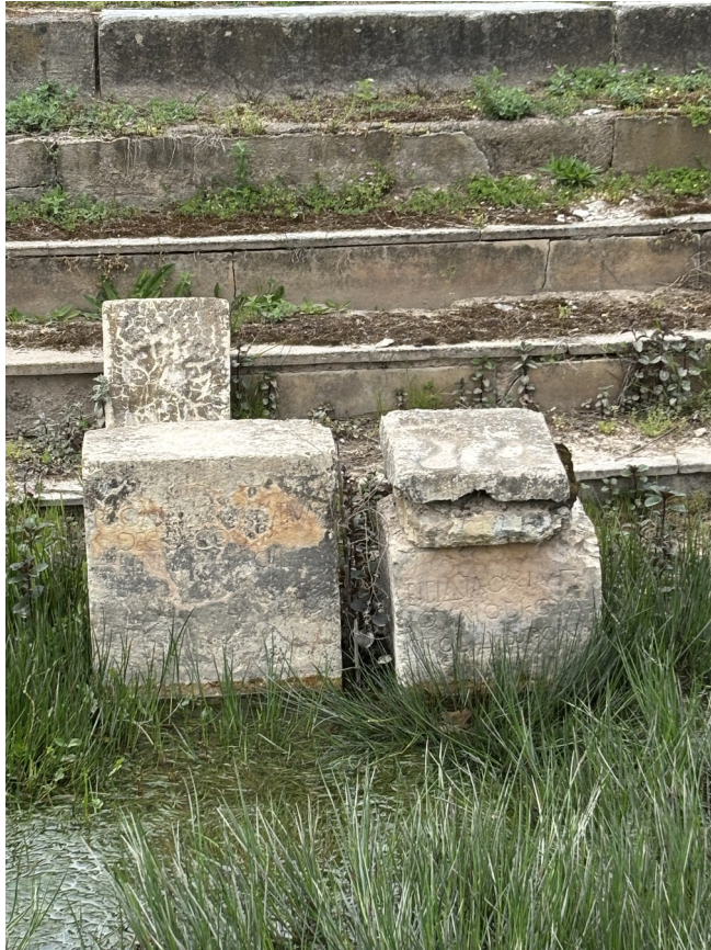
Figure 4: Deterioration of the surface of inscribed columns (May 2026, personal archive).
