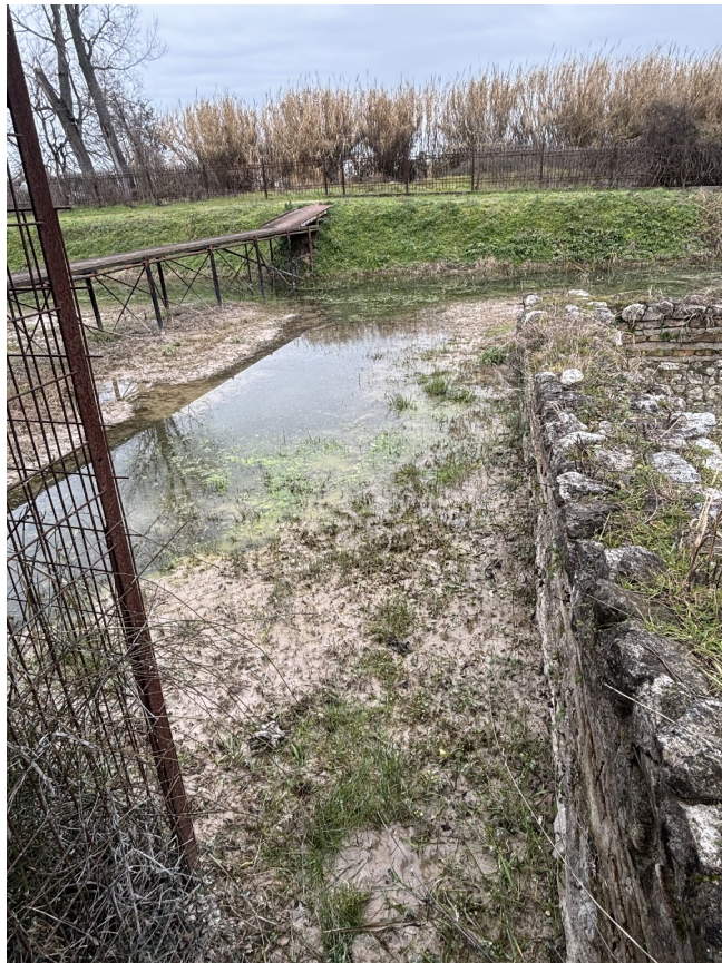
Figure 4.39: Intensive presence of groundwater and mud at the Dionysos villa (personal archive).
