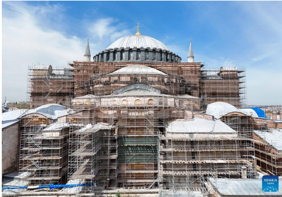
Figure 24. Photo taken on April 14, 2025 shows Hagia Sophia under restoration in Istanbul, Türkiye. Türkiye on Monday started the first-ever comprehensive restoration work on the main dome of Hagia Sophia, one of the most important historical sites in Istanbul. (Xinhua/Liu Lei)
