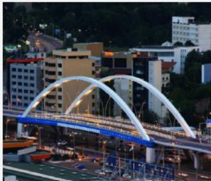
Arch Bridge - Basarab - Bucharest
