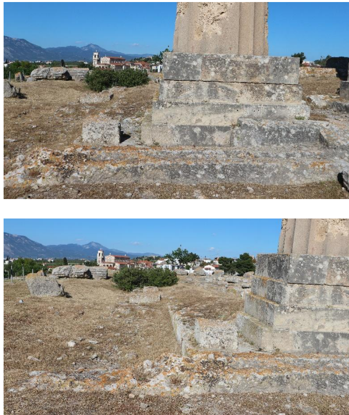
Figure A.86-94. General condition of the stepped foundation platform (krepidoma).
