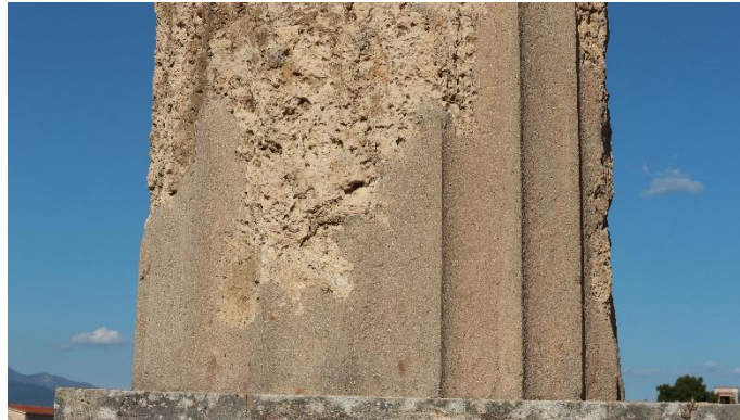
Figure A.7-14. State of preservation of Column 1 (C1), front elevation.
