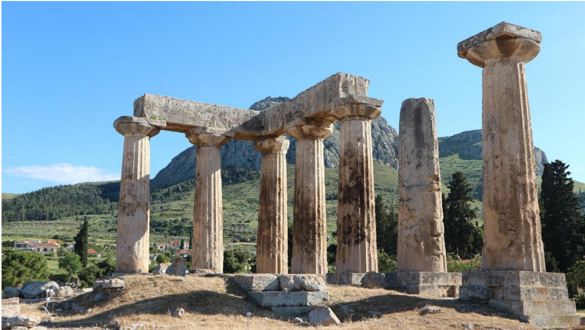
Figure A.3. Overall condition of the surviving columns and architrave, viewed from the interior.
