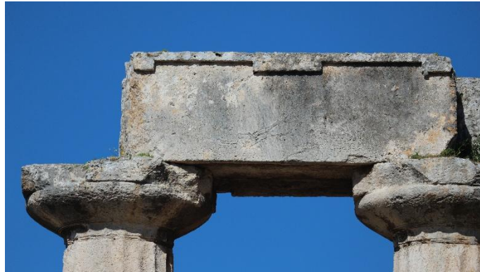
Figure A.4-6. General condition of the architrave and adjacent Doric capitals.
