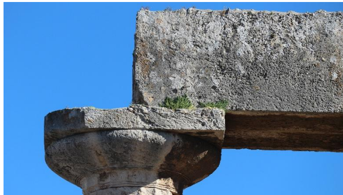
Figure A.82-85. General condition of the architrave and adjacent Doric capitals, viewed from the interior.
