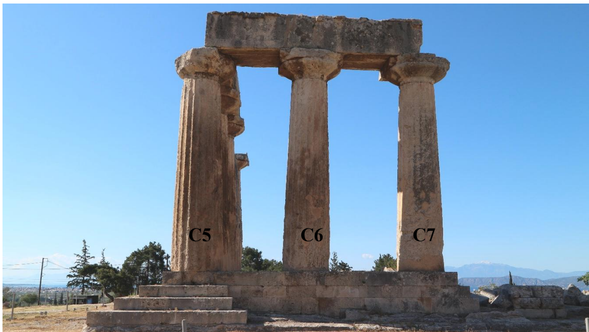
Figure A.2. Overall condition of Columns C5–C7.
