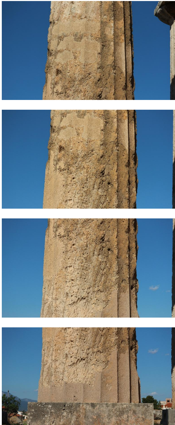
Figure A. 29-37. State of preservation of Column 4 (C4), front elevation.
