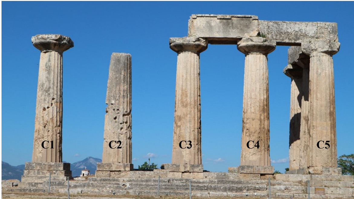
Figure A.1. Overall condition of Columns C1–C5, front elevation.
