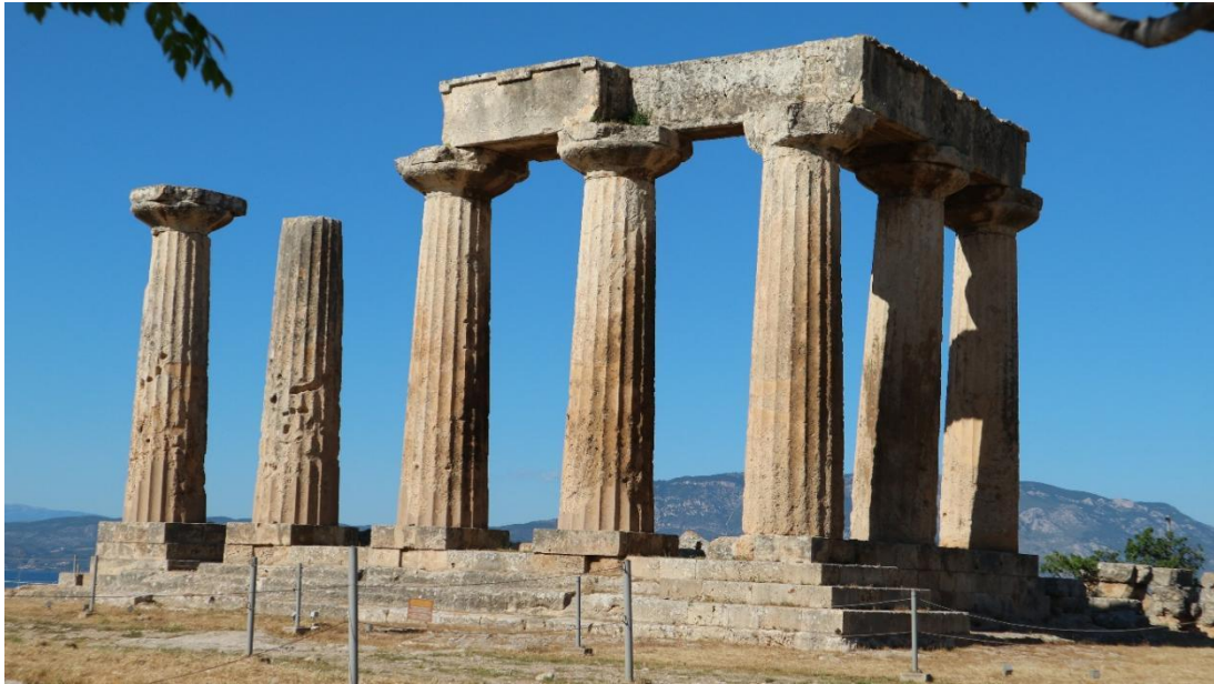
Figure 24. Apparent outward inclination of the columns on the three-column side of the Temple of Apollo.
