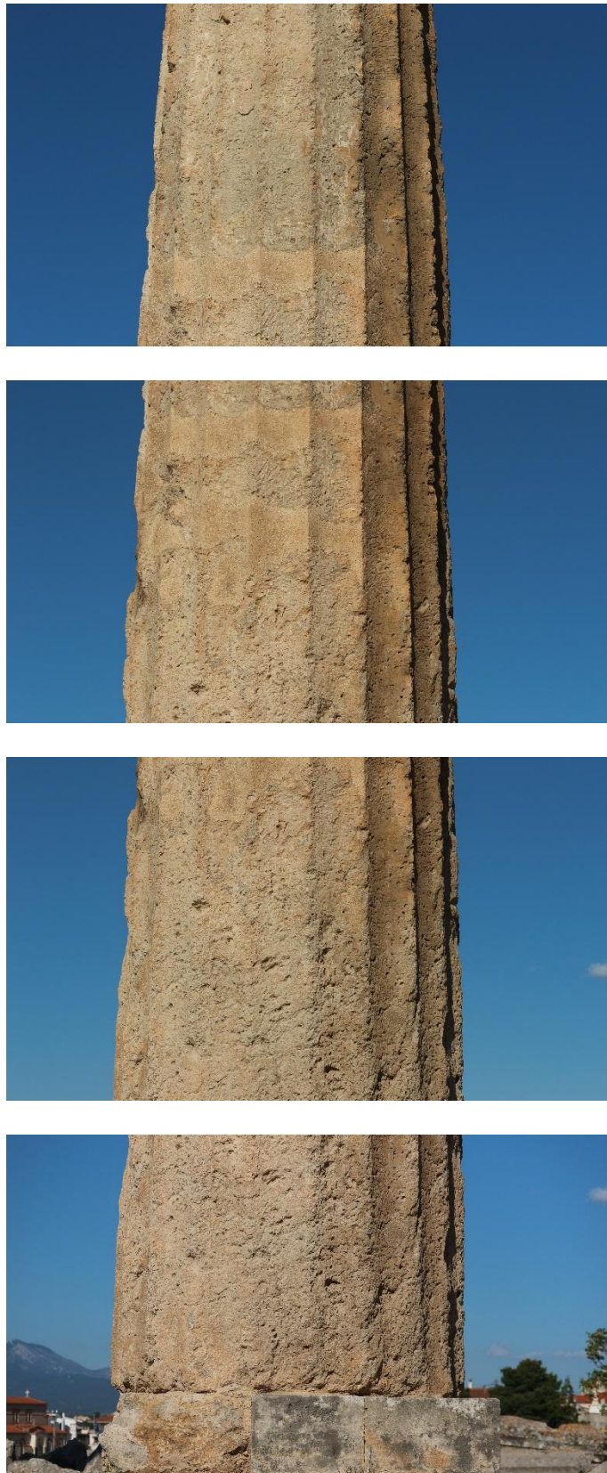
Figure A. 38-45. State of preservation of Column 5 (C5), front elevation.
