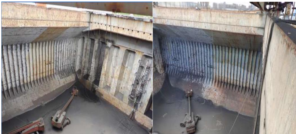
Figure 15 Sand blasting in cargo holds
