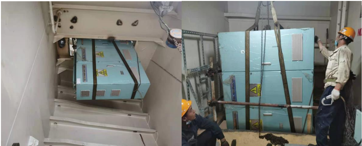
Figure 25 UV power supply panel installation
