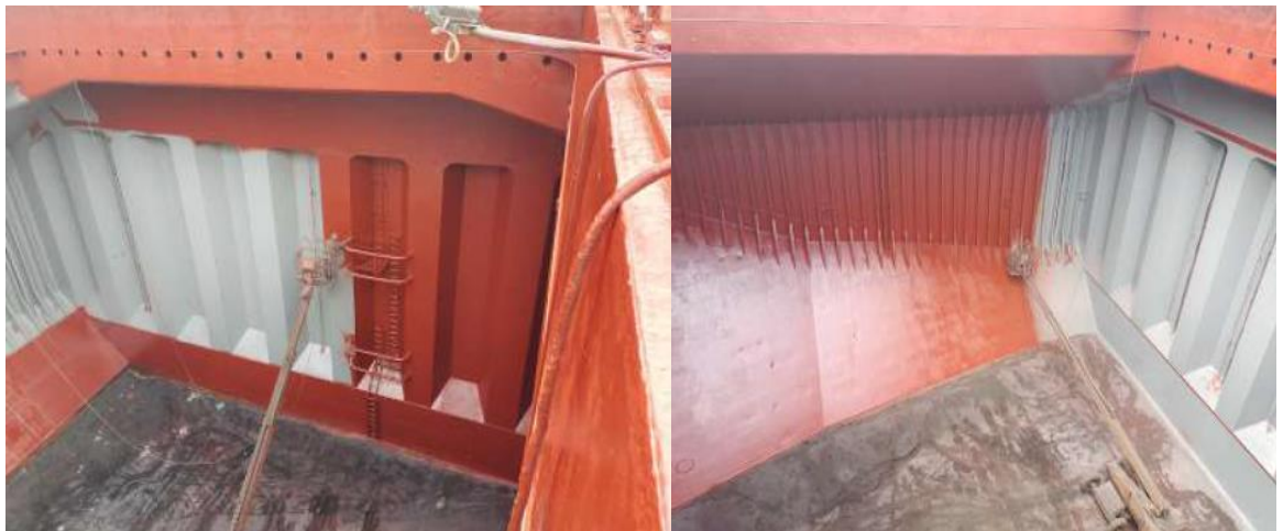
Figure 17 Apply 2nd coat in cargo holds
