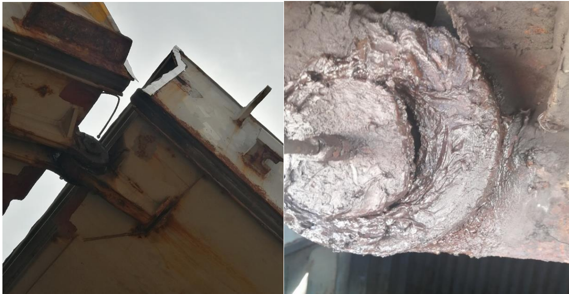
Figure 13 Intermediate hinge pin rotation with stopper plate damaged.
