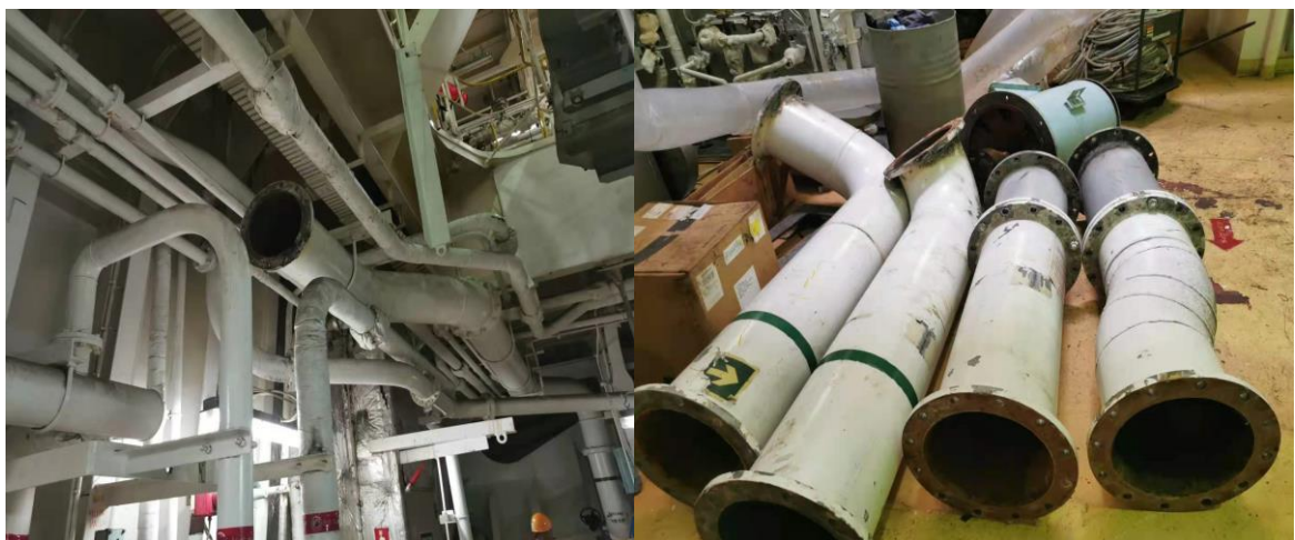
Figure 23 BWTS old pipes dismantle
